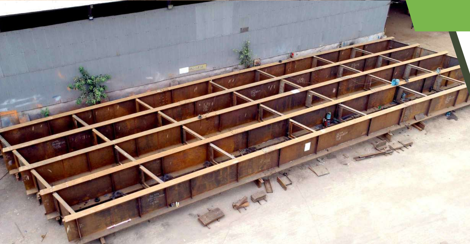
Project : PWD Maharashtra Girder Type : ROB Composite Girders Span : 30 M X 8
